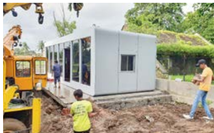
↑ Chira slabs (right) are made of compacted red mud found in the Konkan belt and are a substitute for marble → An Olle Pod being anchored to the Earth with cranes. It is 480 sq ft in total and can be transported anywhere
